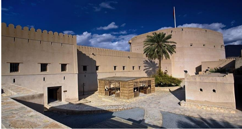
Figure 3: Traditional Omani constructions with thick walls and very limited small screened openings( http://www.muscatdaily.com )
