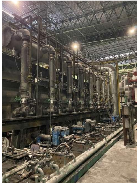
Figure 1. External View of the Reheating Furnace
