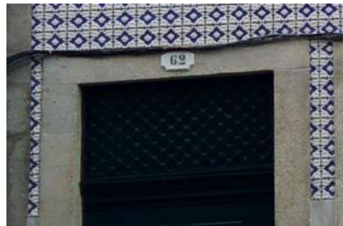
Figure 2: The grid depicted in Figure 1 after treatment and painting of case study
